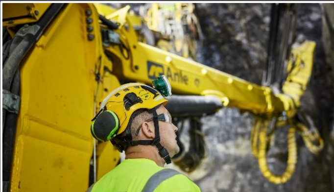
Cable tunnel Sogn-Ulven
