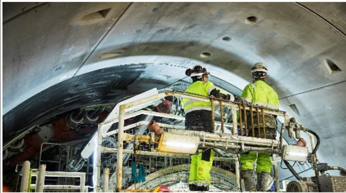
E6 Clean Water Tunnel
